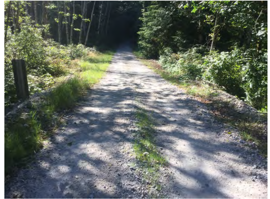
Left Approach Facing Away From Bridge
