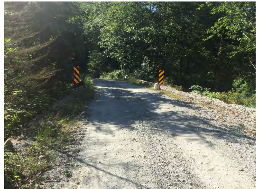
Right Approach Facing Bridge
