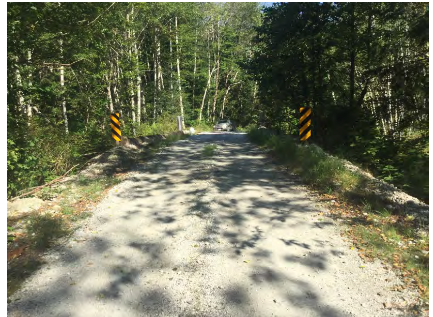
Left Approach Facing Bridge
