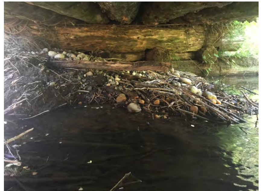
Left Bank Abutment
