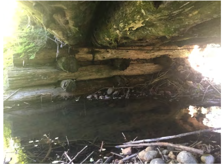
Right Bank Abutment
